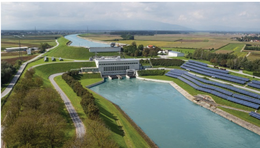
Figure 1: Zlatoličje HPP (photo www.dem.si )
