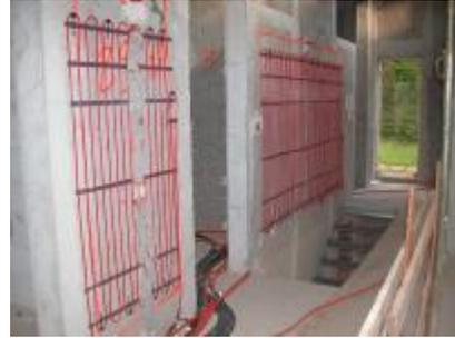
**Figure 14:** Wall heating system
