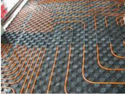
**Figure 13:** Underfloor heating system
