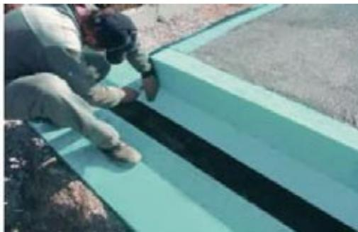
**Figure 6:** Placing of XEPS isolation
