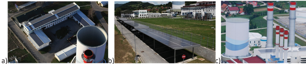
Figure 2: Photovoltaic systems MFE TEB 1-3
