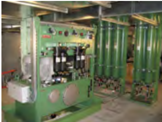
Figure 5: Typical Hydraulic power unit for Saxo turbine.
