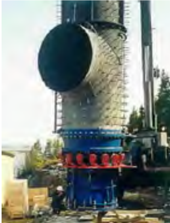
Figure 3: HPP Pouvoir Riverin: The factory-preassembled part that includes inlet elbow, stay vanes and guide vanes with regulating mechanism is ready for concreting in one piece.
