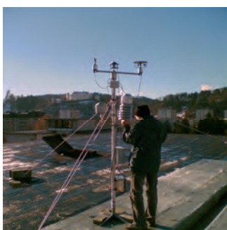
Figure 1: Establishing the mobile meteorological station on a high school roof (Korošec, Tržan, 2006.)
