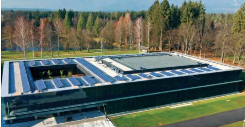
Figure 2: Protocol and congress centre in Brdo pri Kranju with a 43 kWp solar power plant
