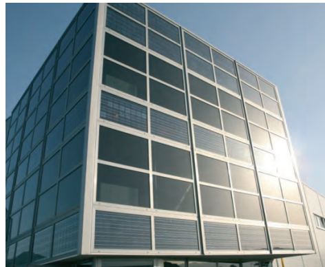
Figure 3: The facade of the headquarters of the company BISOL, d.o.o. - the first facade in Slovenia with built-in photovoltaic modules
