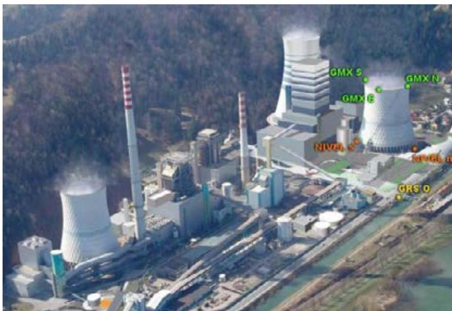
**Figure 6:** The position of the measuring points of the automatic uninterrupted GNSS monitoring in TEŠ.
