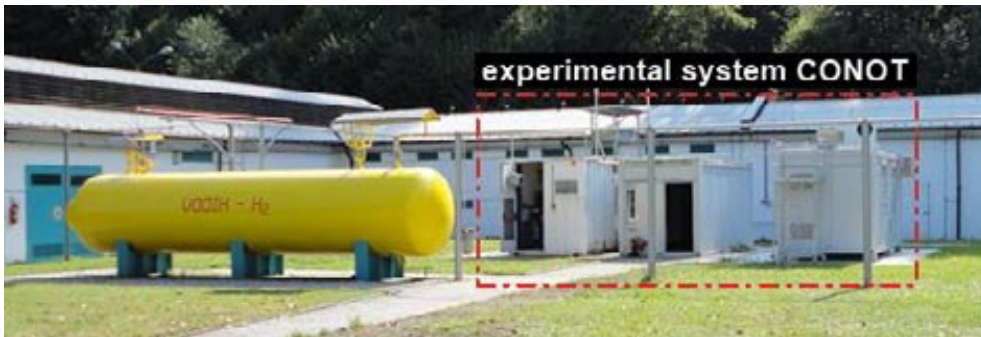
Figure 5: Photograph of the outside of the hydrogen technology testing facilities
