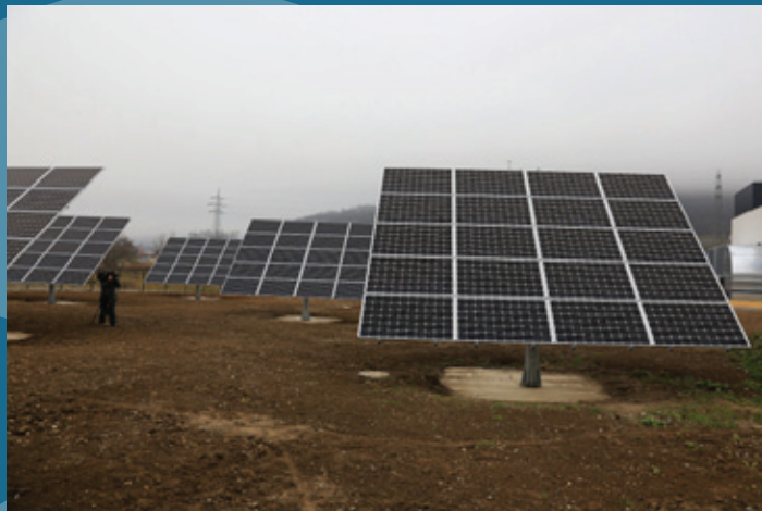
new photovoltaic field at the Institute of Energy Technology
