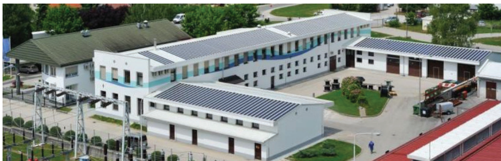
Figure 1: The office building
